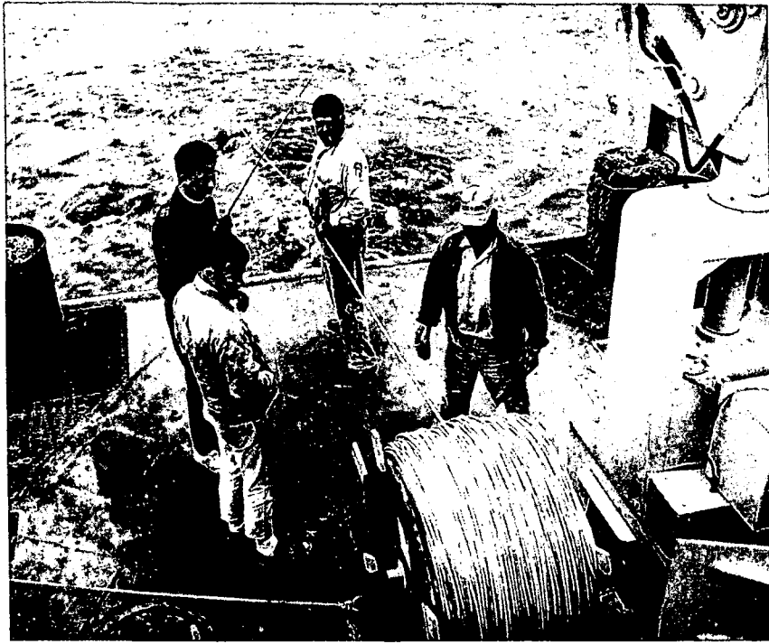
Figure 16. Spooling out the nylon mooring line.
