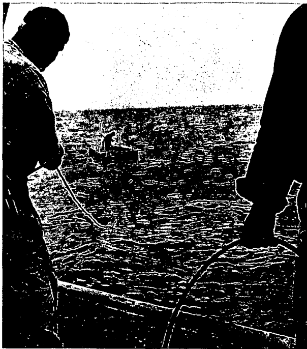
Figure 15. Laying of the instrument cable.
